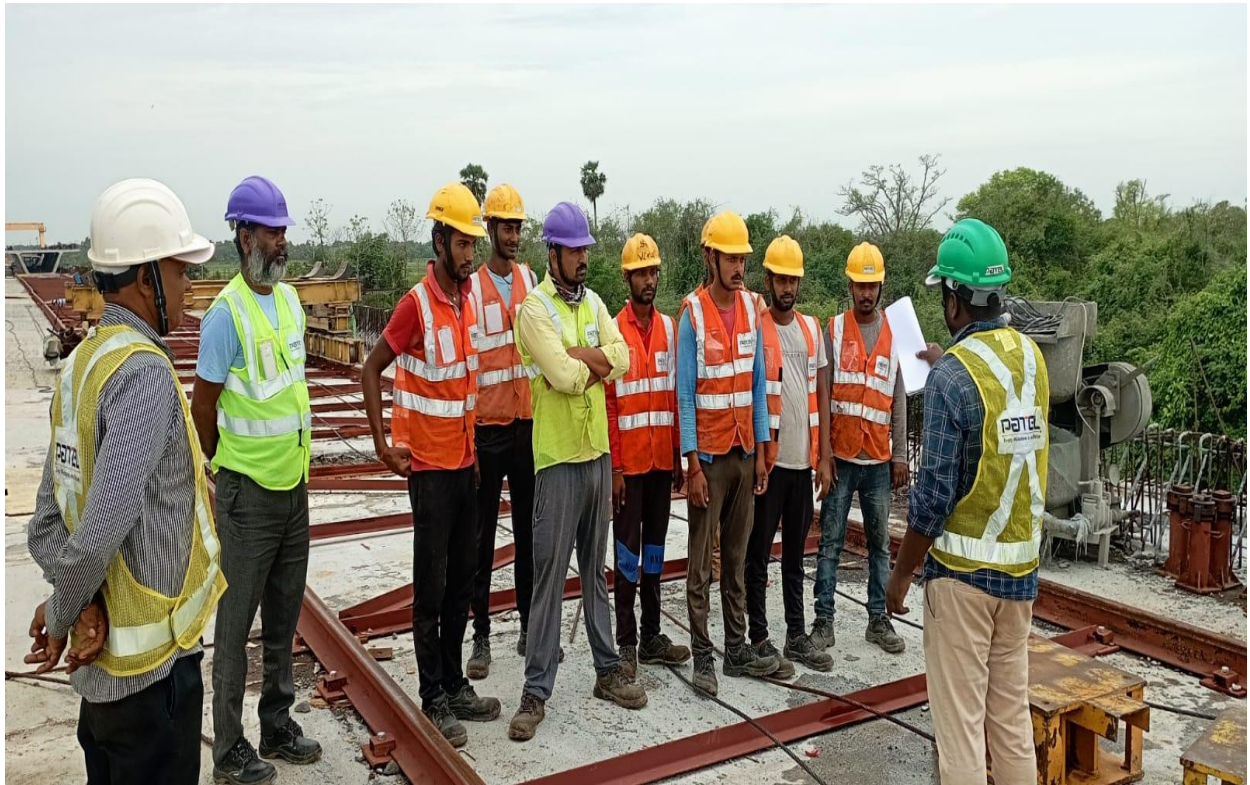
Safety instructions given to labours at Ch. 107+400 (Major bridge)
